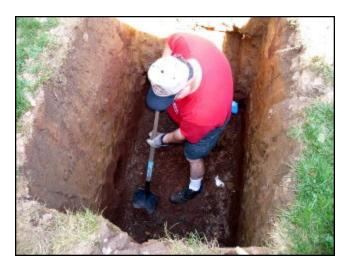
squaring off the bottom of the hole by hand with a shovel.
